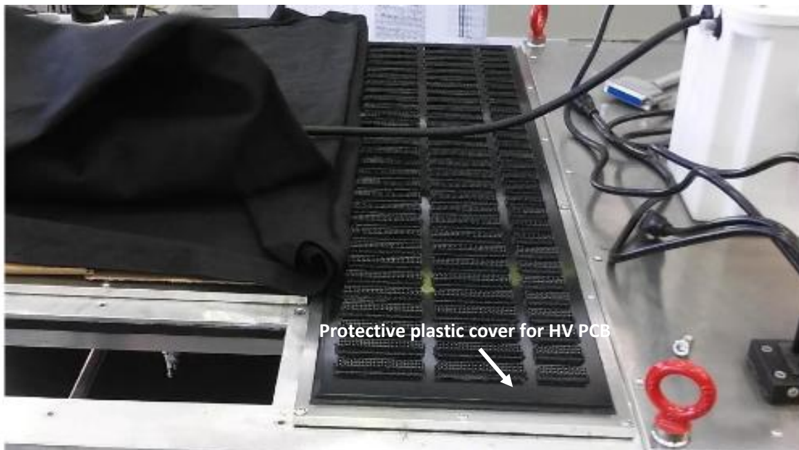
High voltage PCB installed in NPS detector frame with plastic protective cover
